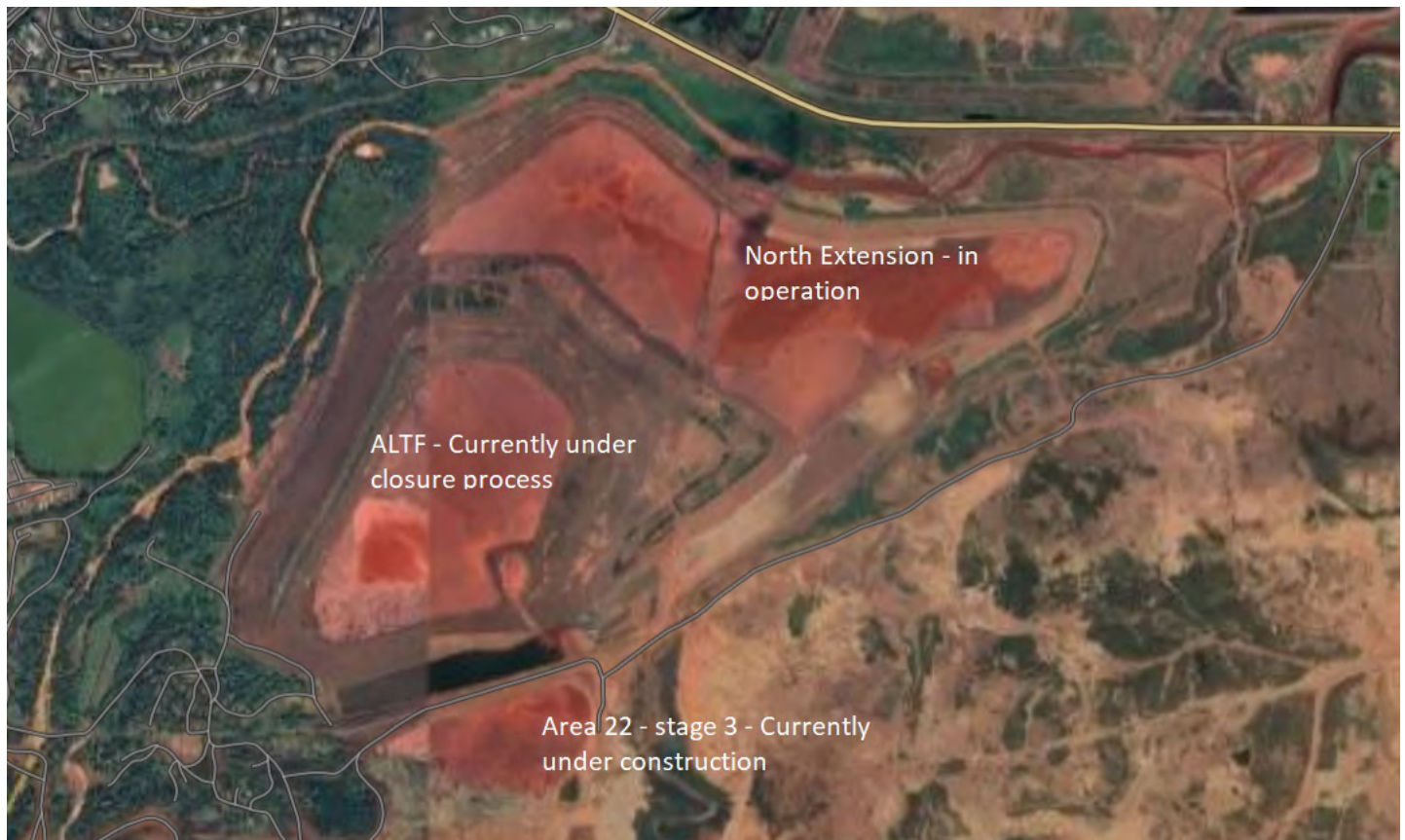
Figure 2: Tailings Management Facilities
